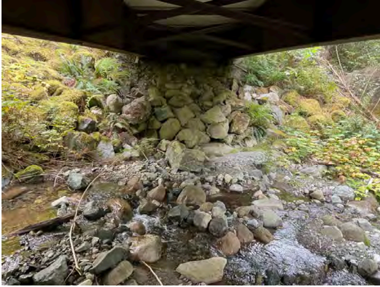
Left Bank Abutment when facing downstream
