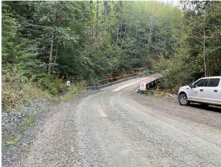
Approach from Right Bank when facing downstream
