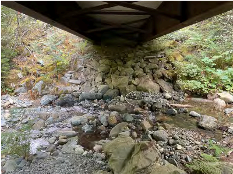
Right Bank Abutment when facing downstream
